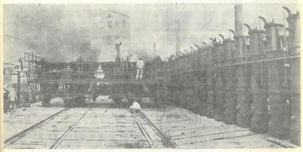
Coke oven being charged with high-caloried coal and ore powder NEW KOREA No. 29, 1958 that of the high-caloried coal. And on the 20th of the same month the whole oven began to produce the ferro-coke. Throughout the first stage experiments, the research personnel worked with the workers helping them in every way.
