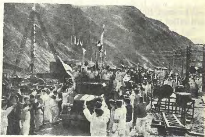
Young socialist builders, volunteers from all parts of the country, have come to undertake the construction of the Kangge Power Station
