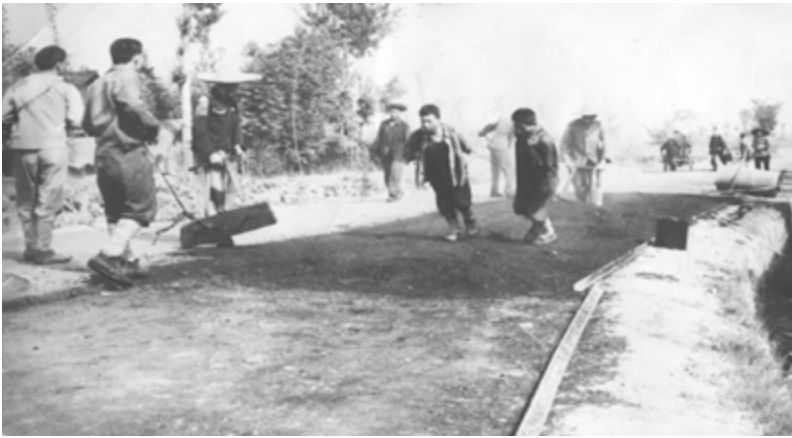
Figure 3. Building a road for a Third Front factory. Source: “‘三线文化’ 三线建设部分老照片选登” [“Third Front Culture”: Select Published Old Photos of Third Front Construction]. 每日头条 [Meiri Toutiao], 20 August 2017, available online at: kknews.cc/zh-cn/news/a8jbqa6.html .
