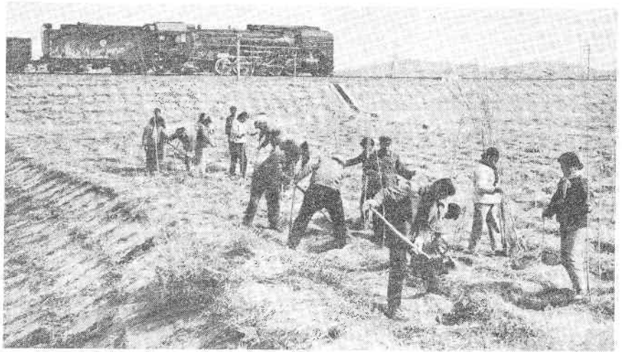
Along the Baotou-Lanzhou railway, grass is planted in checkerboard grids to give new seedlings protection from the wind. Xinhua
