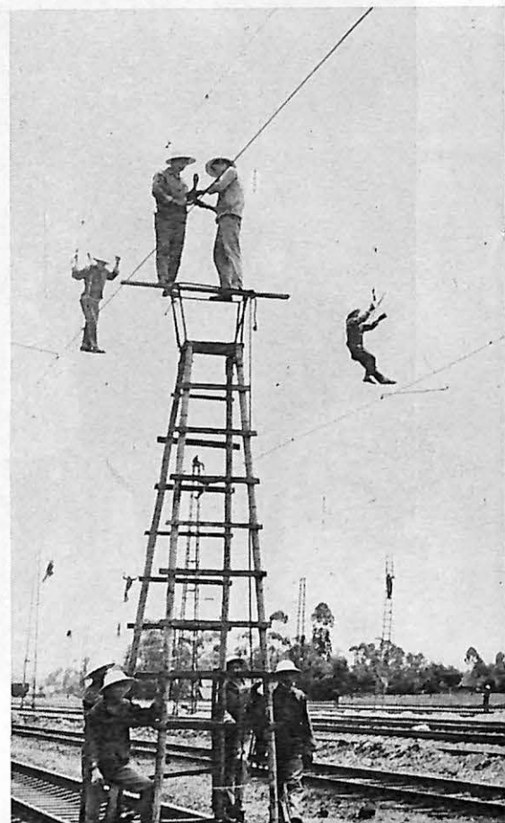
Work on an overhead line.
