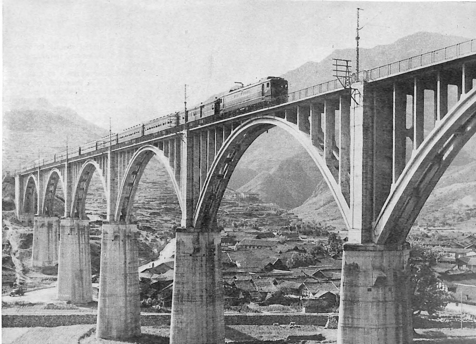
A China-made "Shaoshan" electric locomotive pulls a passenger train along the line between Paoki and Chengtu.
