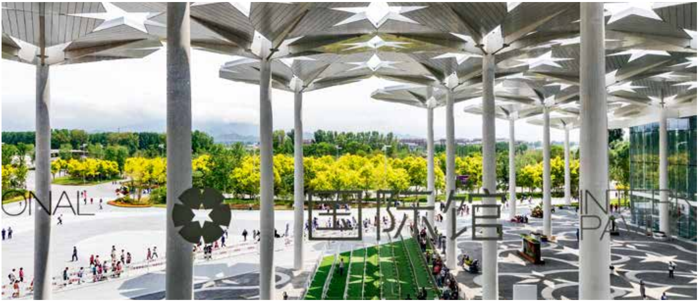
The shade umbrellas outside the International Pavilion double as rainwater collectors.
