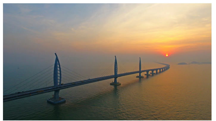
The aerial photo of Hong Kong-Zhuhai-Macao Bridge taken on December 31, 2017 (XINHUA)
